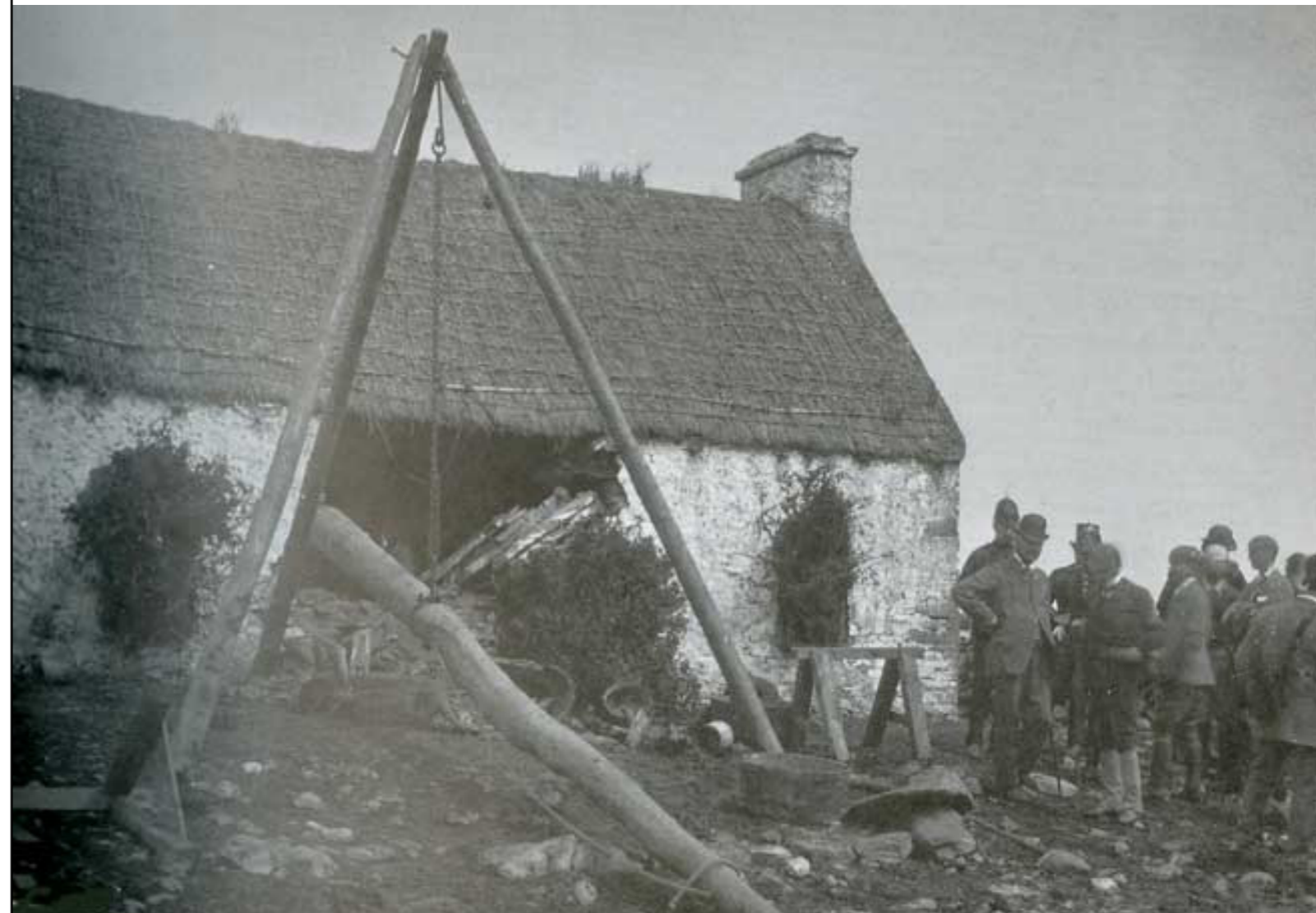
v Figure 8 Example of a battering ram being used to demolish house walls in order to effect an eviction of its inhabitants. Often, several of the walls were knocked in and the thatched roof was torn off, sometimes being set on fire, making the house uninhabitable. Photo courtesy of the National Library of Ireland.
